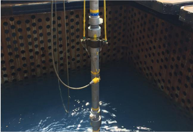
**Cementing:** Two techniques were available to place the cement plugs as per the applicable regulations; punch and squeeze or pump and pull. The client's preference, based on assurance of the optimum quality, was to employ the pump and pull technique.
