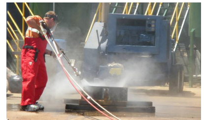
Ultra High Pressure Cleaning
