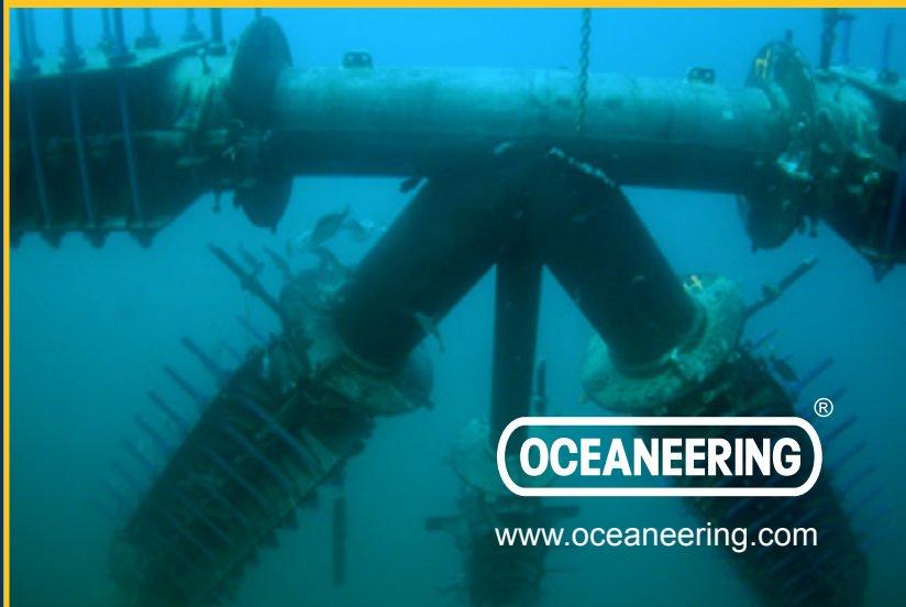
Stress Grouted Structural Repair Clamps
