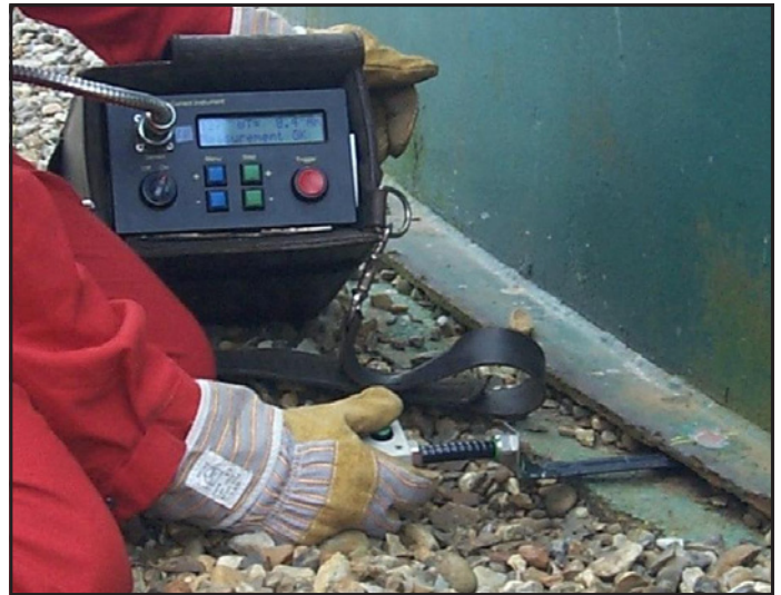
Storage Tank Inspection: Inserting PEC probe into the gap between the annular ring and tank base is a simple operation and can be performed with the tank in service.
